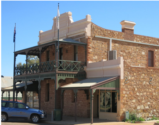
Above: The Shire of Cue has a rich history reflected in its built heritage preserved along the Main Street
