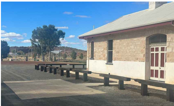
Railway Building The Railway Building is now accessible. The next stage is footpath construction from Wittenoom Street.
